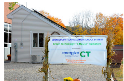
Wolcott Tech E-House.
