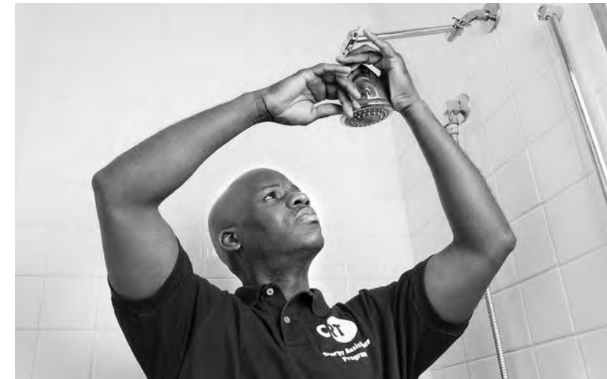
Low-flow shower heads save water and associated heating costs.
