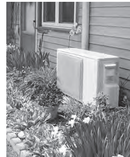
The outside unit of the ductless heat pump is quiet and has a small footprint.
