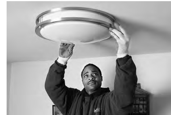
WRAP technicians install energy-efficient ceiling fixtures for the Portland Housing Authority.
